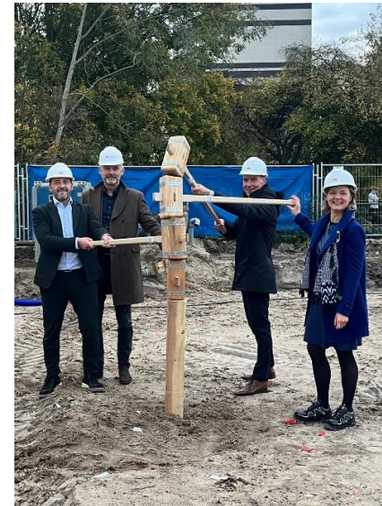
Start sloop-herstructurering Havezate te Zwolle
